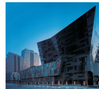
SOHO Shangdu, Beijing
